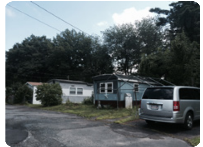
19% of MH is anchored to the ground by a masonry foundation. 1
